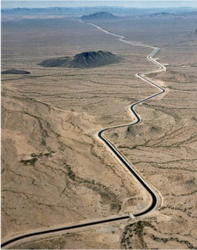
Figure 10.2: Central Arizona Project canal.
